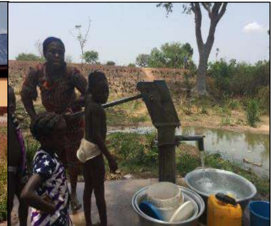
Rehabilitation of borewell pumps
