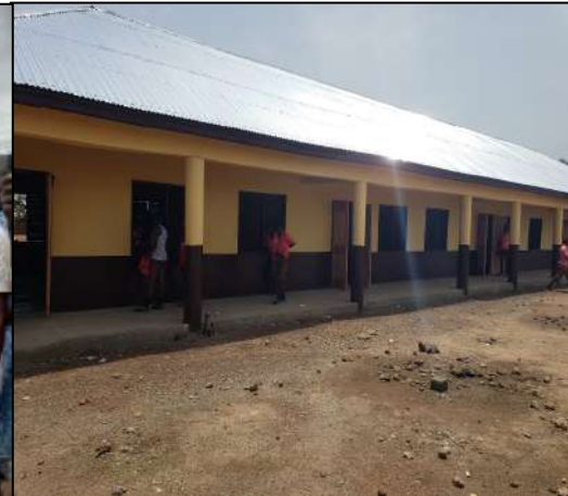
School building renovation
