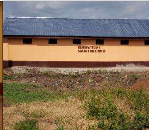
Rehabilitation of public toilets
