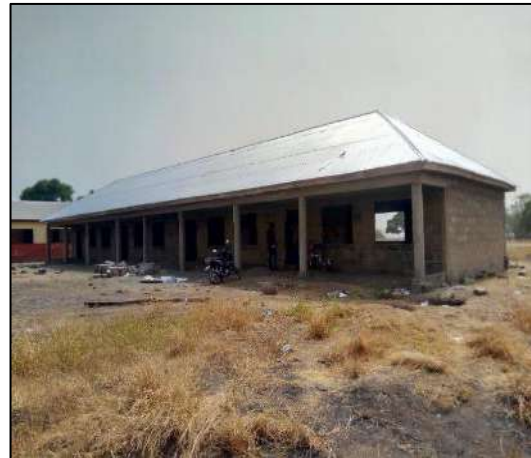
Construction of teachers housing unit
